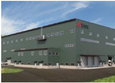
Epson Atmix has begun construction of its new recycling facility (Courtesy Epson Atmix)
