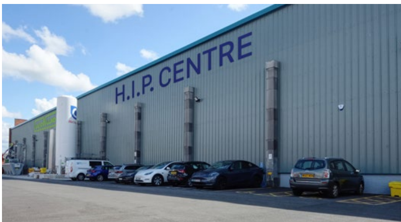
Wallwork Group has established a new £10M HIP Centre (Courtesy Wallwork)
